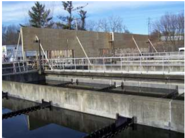
First Wall of UV Building Enclosure
