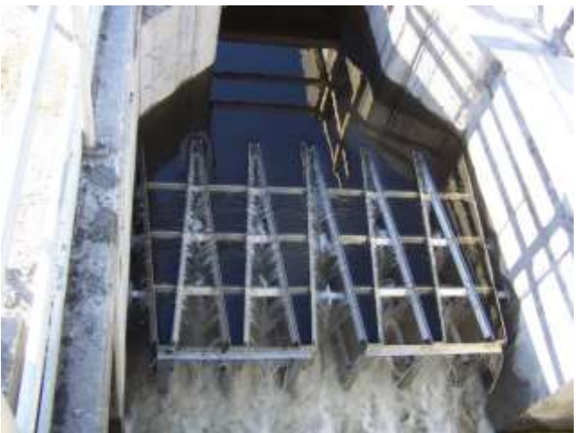
Finger Weirs Control Water Level on UV Bulbs
