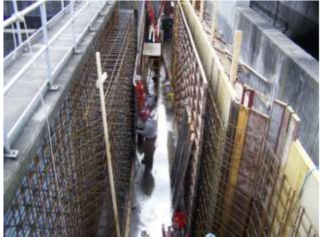
Discharge Channel's Rebar for UV Modules
