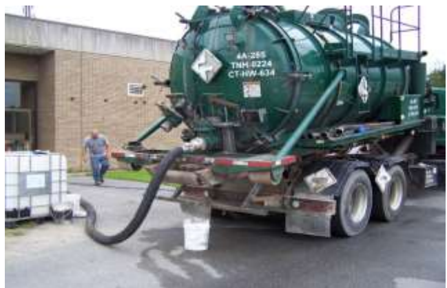
VAC discharging into Sludge & Press Building
